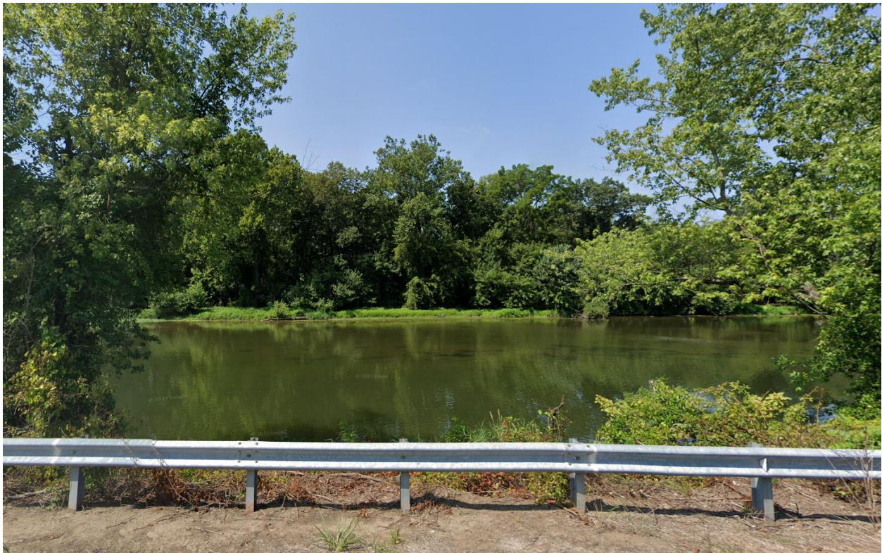
Swatara Creek Google Street View
